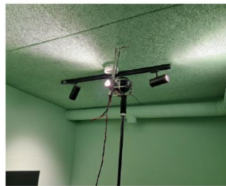
Figure 6b: Green ceiling.
